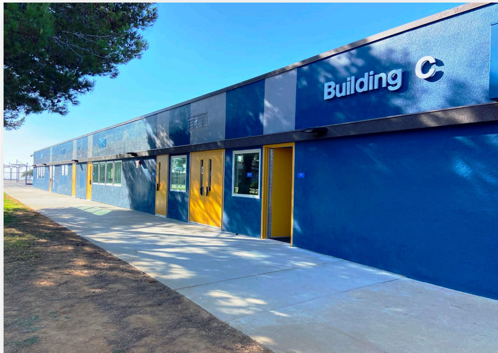
OCMS-Bldgs. C & I Modernization
